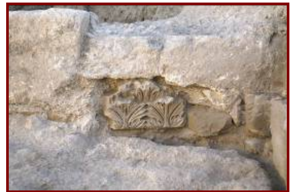
Figure 11: Capital of a Corinthian pilaster integrated into the back wall of the eastern shop.
